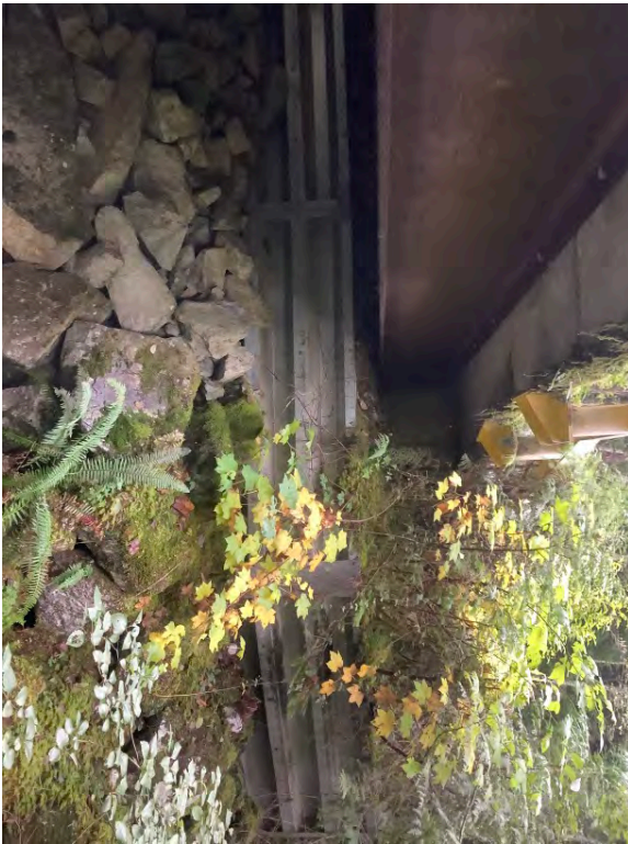
Left Bank Abutment when facing downstream
