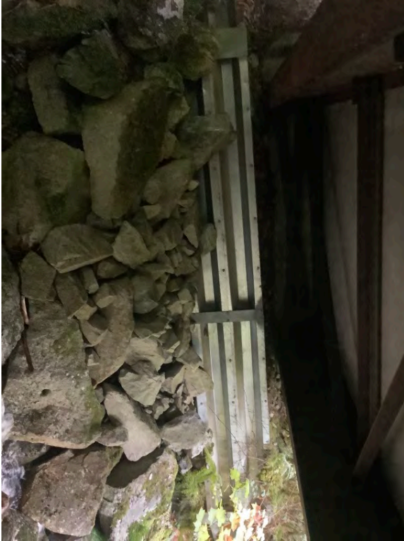
Left Bank Abutment when facing downstream
